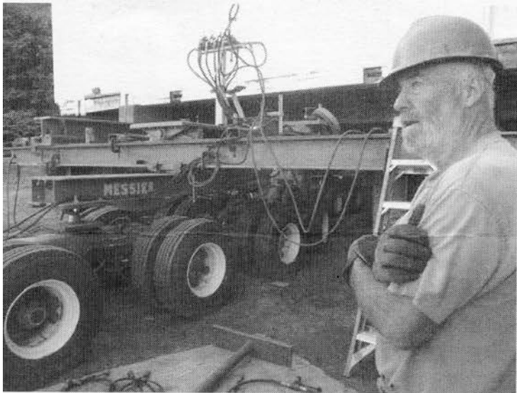
Norm Messier stands beside the Grammar School, mounted on three wheeled carriages, ready for the move. Norm's son Jason and a small experienced crew packed the building up in June, and removed the granite foundation stones from underneath. Messier's Moving Company delivered them to a granite shed in Barre, where they were cut into 3 inch slabs to face the new concrete foundation. Norm's wife Carla sat in front of the building and steered it up the road behind the oxen during the move on August 8. Self powered dollies underneath, donated by Brownie Company Moving, provided power to help the oxen bring the 106 ton building uphill to its new and former home.
