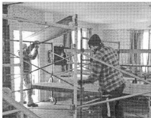
Chris McCarthy and Makaio Maher of Green Timberworks ease the long I-beam through the door.
